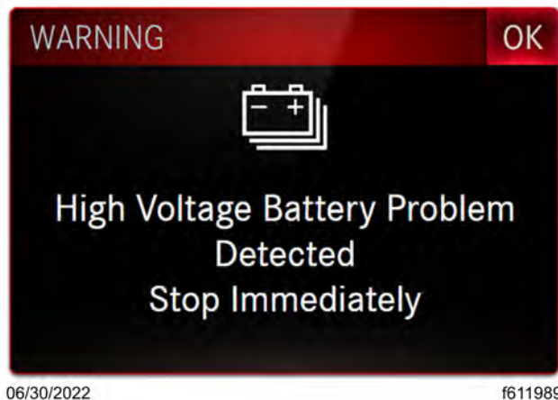
Fig 215, Thermal Event Warning Message
