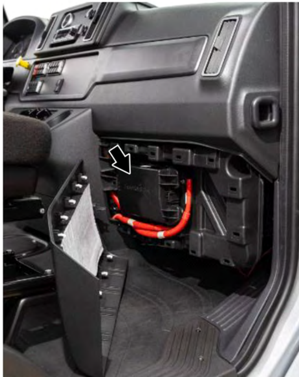
Fig 230, Power Distribution Module (PDMi) Behind Right-Side Dash
